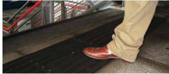
"The purpose of The Corduroy Surface is to warn visually impaired people of the presence of specific hazards; steps, level crossings or the approach to on street light rapid transport (LRT) platforms. It is also used where a footway joins a shared route, it conveys the message "Hazard proceed with caution"
