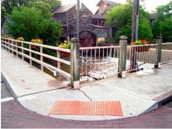
The blister truncated dome as illustrated here is not just extremely durable. It also boasts the benefit of ease of installation and is further complimented as a more aesthetically pleasing product than its fiberglass or resin counterparts. When installed, Visul's detectable warning system benefits from the stone blend giving the appearance of natural brick.
