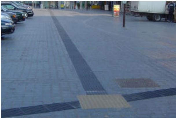
A combination of different warning and information surface tiles has been used in Belgium to assist blind and partially sighted students in finding their way safely from school to the local shop and back. Blister surface is used to indicate roadcrossing points and guidance tile is used to provide a detectable path across an open plaza to the shops.
