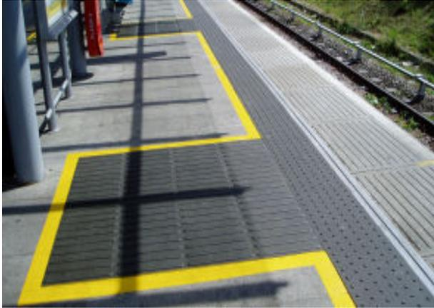
The guidance tile has been used to great effect on Docklands Light Railway London. The driverless trains on DLR come to a pre-determined stop position; the guidance tile is used to indicate the position of the train doors and therefore allow the visually impaired to prepare for the train's arrival and make a safe entry into the carriage.
